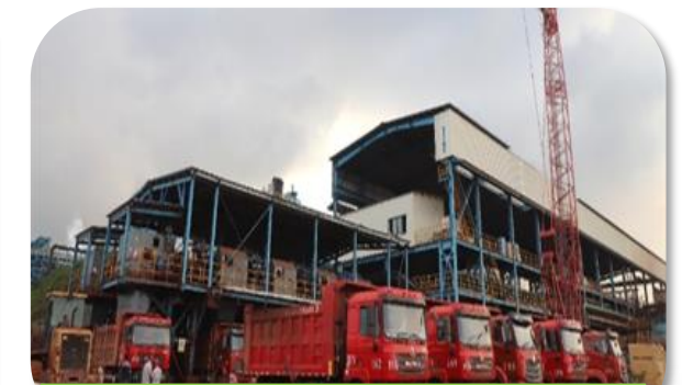
TAILINGS FILTER PRESS WORKSHOP
